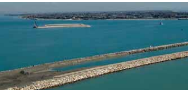
3. Malamocco inlet. The outer breakwater and the construction of the lock for large ships
