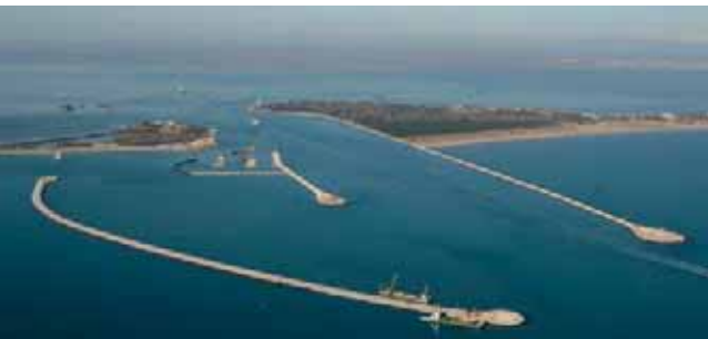
4. Chioggia inlet. The refuge haven and locks
