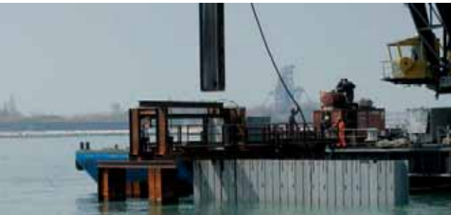
5. Chioggia inlet. Construction of the locks
